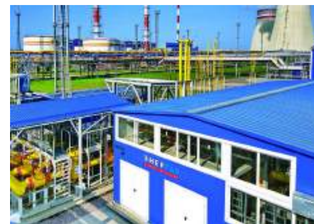
ENERGAS fuel gas treatment station for Pregolskaya TPP in Kaliningrad
