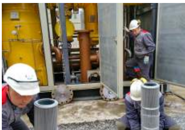
Local repair of the gas booster unit directly at facility
