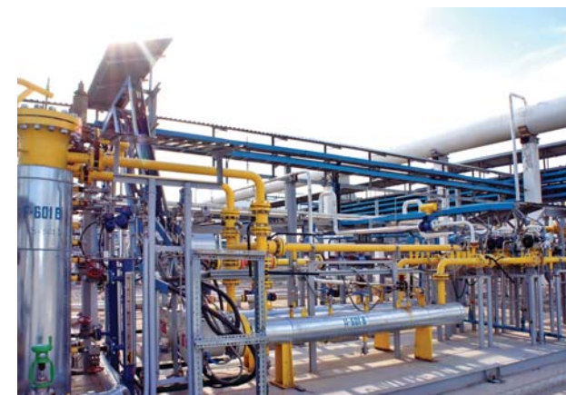
Photo 6. Fuel and starting gas treatment system for BCS Alan (Uzbekistan). Electric gas heaters are used here
