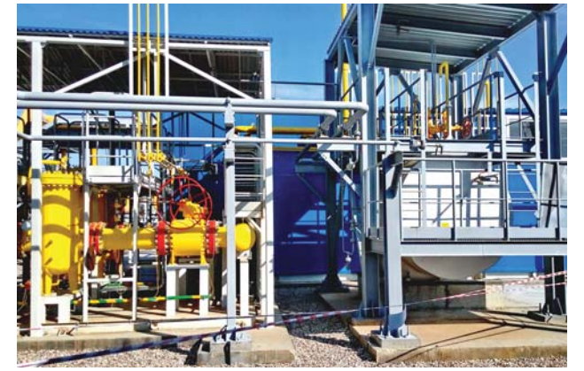
Photo 3. External pre-filtration module and condensate drainage module
