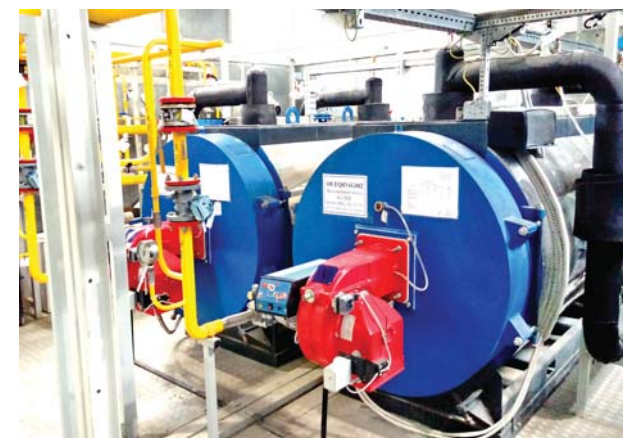
Photo 7. Compartment of block-type boiler room is integrated into common process module
