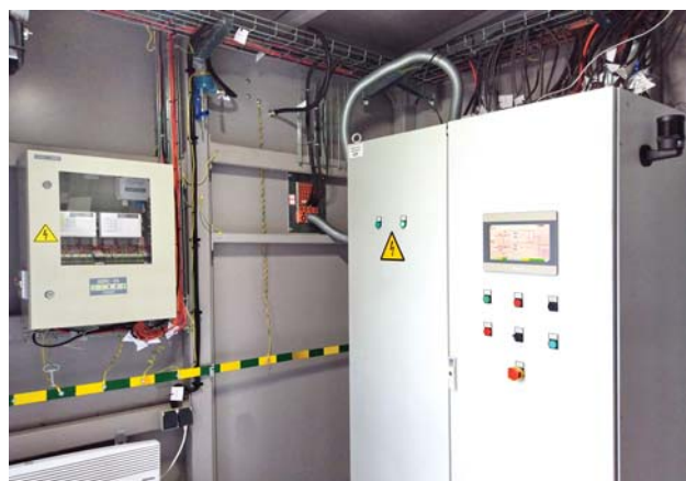
Photo 5. ACS compartment of complete gas treatment unit
