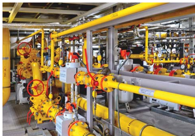
Photo 4. Commercial gas-metering unit with ultrasonic flow meters
