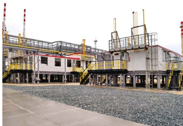
Photo 8. Multi-packaged fuel gas treatment facility for the facilities of CGCTP at East Urengoy – the main (on left) and standby modules
