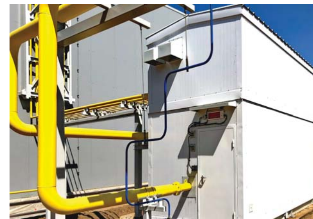
Photo 11. Block-type gas purification unit for GTU-TPP in Yelabuga is a compact unit in the basic configuration
