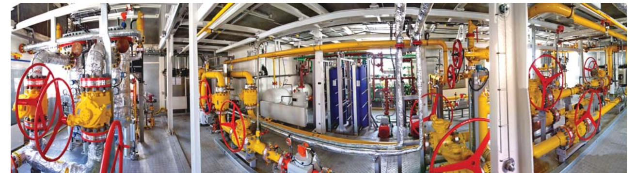
Photo 2. Separate block-boxes during erection create a common process space of a multi-packaged unit (panoramic view)
