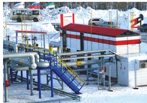
Photo 10. Associated gas treatment unit for the GTU-CHPP at Usinsk field of LUKOIL-Komi
