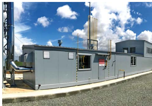
Photo 9. Automated gas distribution station manufactured by ENER GAS Group
