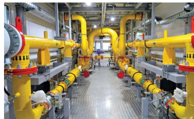
Photo 13. Gas-control station will provide fuel for the direct oil heating furnaces at oil treatment plant Usa-Heavy Oil
