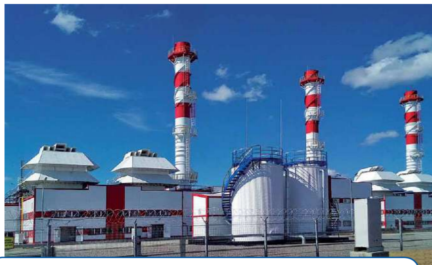
Photo 1. Usa power supply complex – GTU-CHPP with an electric capacity of 100 MW
