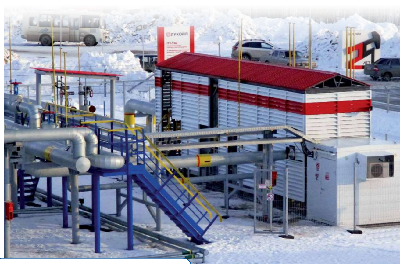
Photo 3. ENERGAS associated gas treatment station
