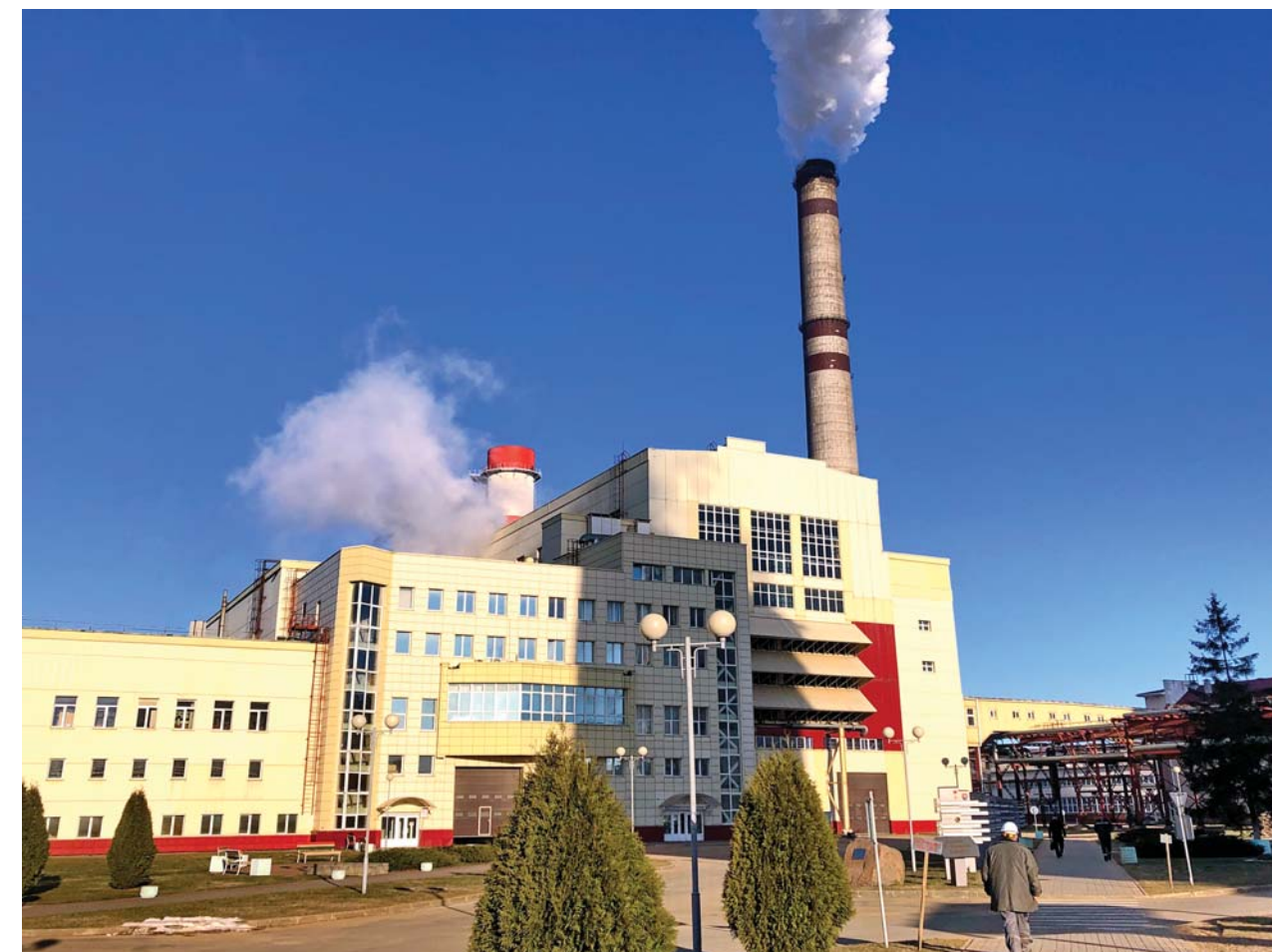
Photo 1. CCGT-230 combined-cycle plant at Minsk CHPP-3
