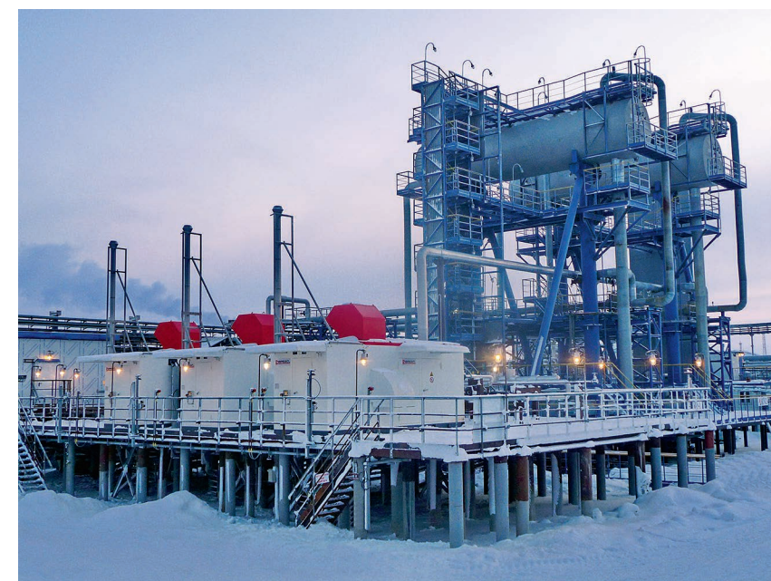
PHOTO 1-2. Varandey field (LUKOIL-Komi). Oil treatment plant and ENERGAS low pressure gas compressor station
