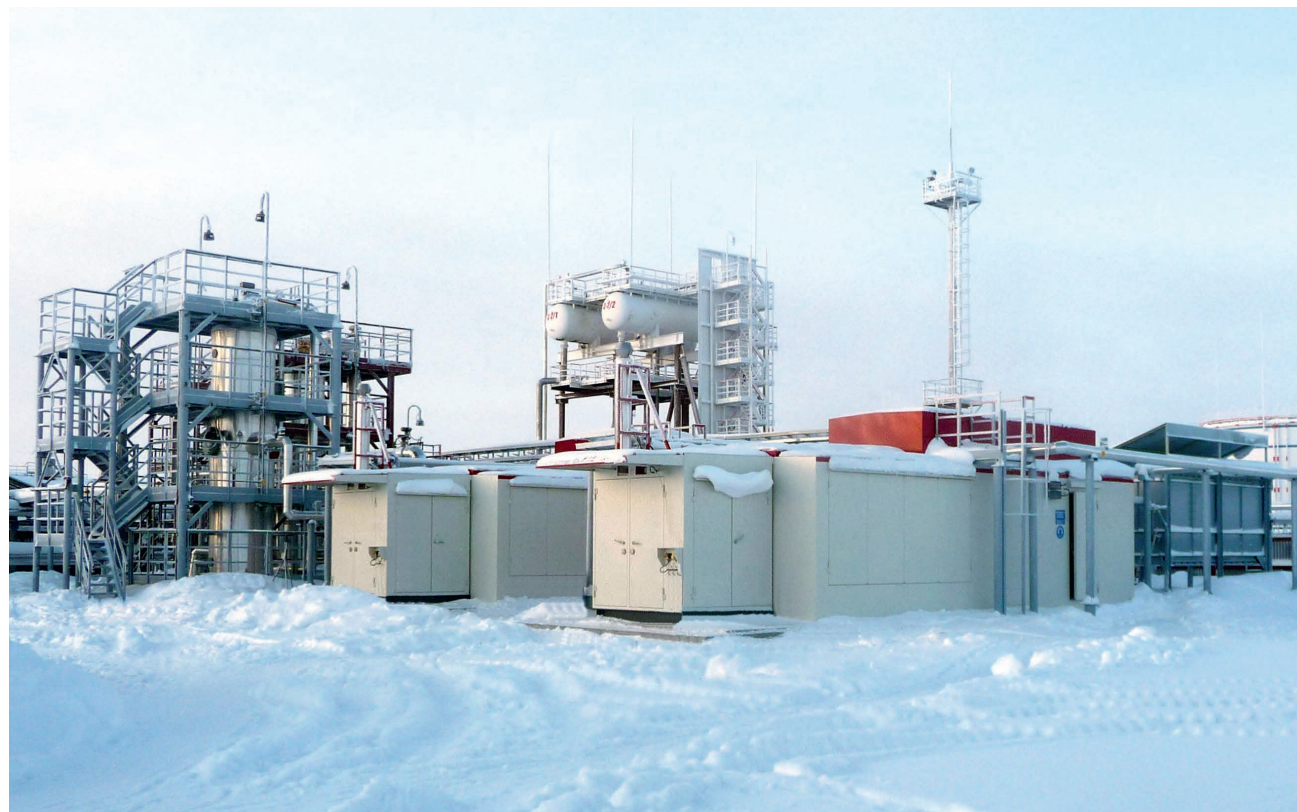
PHOTO 7. Arctic version CUs compress LP APG as a part of North-Labatyugan field compressor station of low separation stages (Surgutneftegas)
