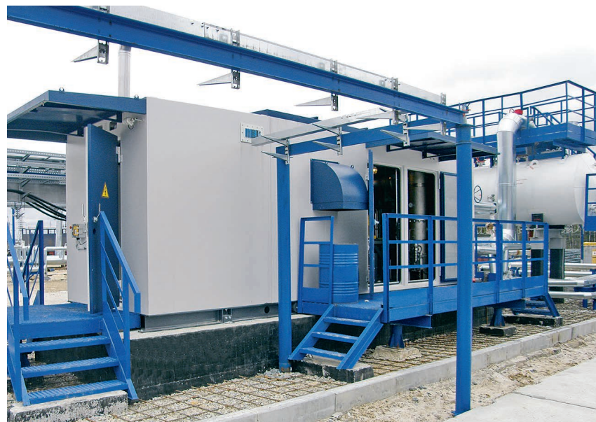
PHOTO 4. ENERGAS vacuum compressor unit at BPS-1 of Vyngapur field (Gazpromneft-NNG)
