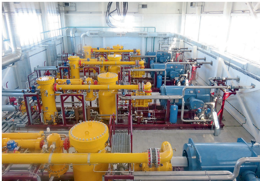
PHOTO 6. Compressor station of the hangar (intra-shop) type for the East-Messoyakha field GTTP
