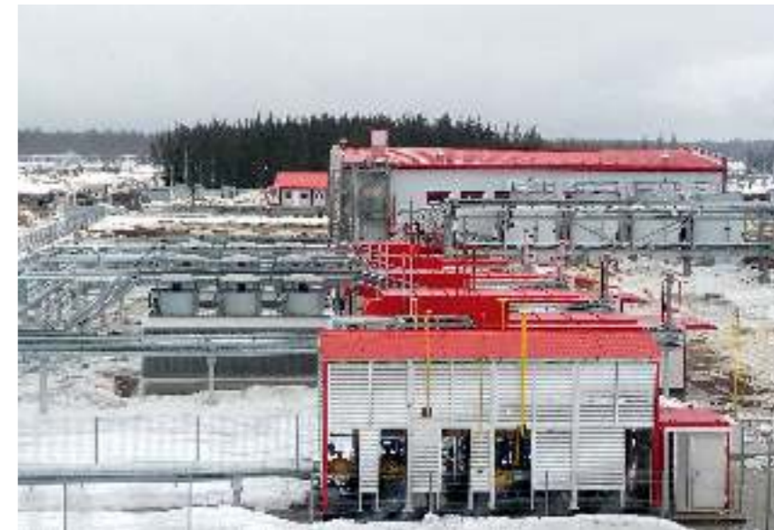
PHOTO 8. Gas treatment system of ENERGAS at the Yarega oil-and-titanium field
