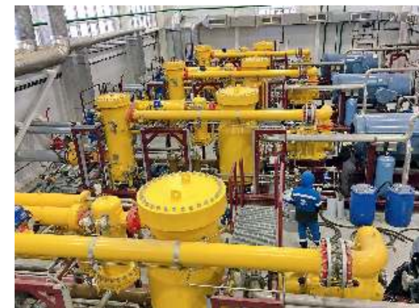
PHOTO 4. Fuel gas treatment facility for the GTPP at Messoyakha
