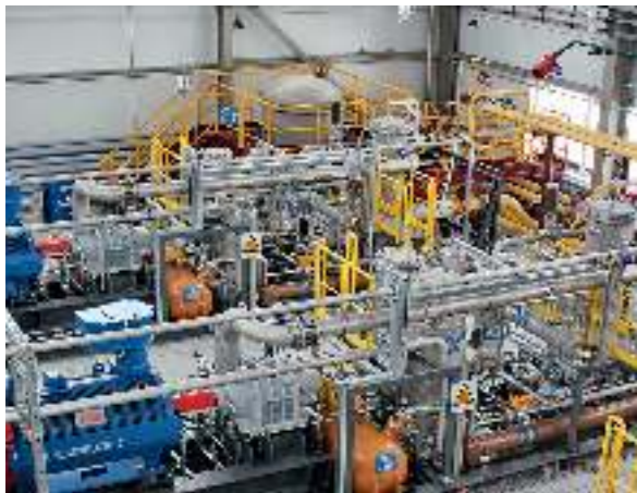
PHOTO 5. BCS of the hangar type as a part of GTPP-24 of the North-Labatyugan field
