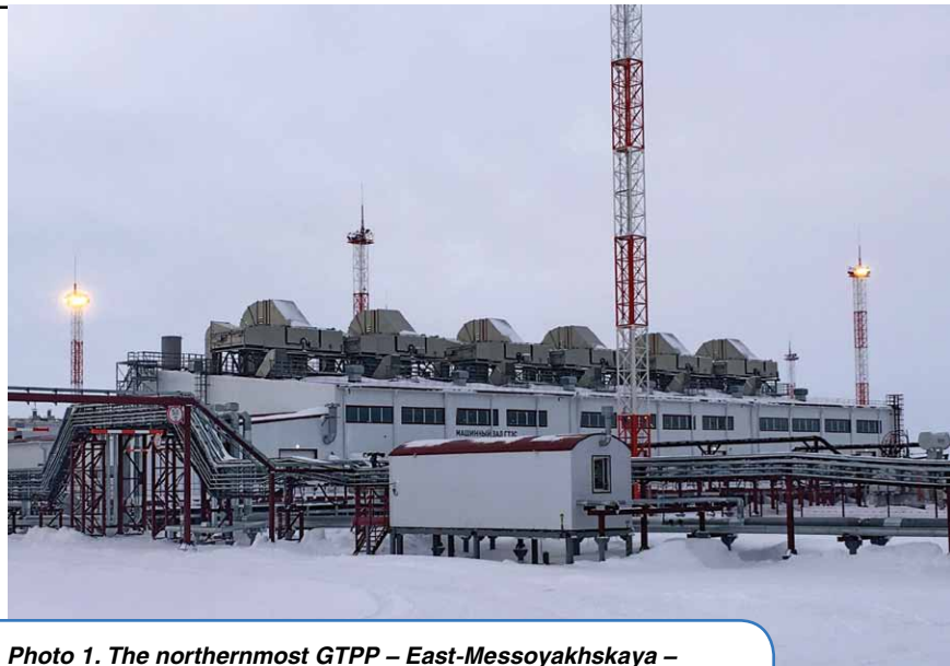
Photo 1. The northernmost GTPP – East-Messoyakhskaya – operates on a low-pressure associated petroleum gas
