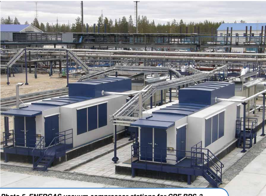
Photo 5. ENERGAS vacuum compressor stations for CPF BPS-3 of Vyngapur field (Gazpromneft-NNG) have a design specialized for LP APG with 0.001 MPa inlet pressure
