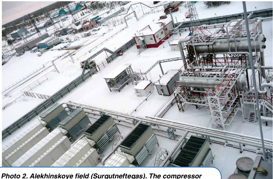
Photo 2. Alekhinskoye field (Surgutneftegas). The compressor station of low separation stages receives APG from several sources
