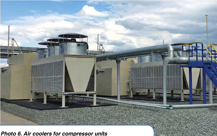
Photo 6. Air coolers for compressor units
