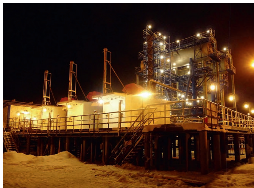
Low pressure booster compressor station on the basis of Enerproject units pumps low-pressure associated gas at the Varandey field of LUKOIL-Komi
