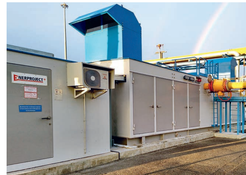
The most powerful Enerproject screw compressor units in Russia provide fuel gas for turbines of the Grozny TPP
